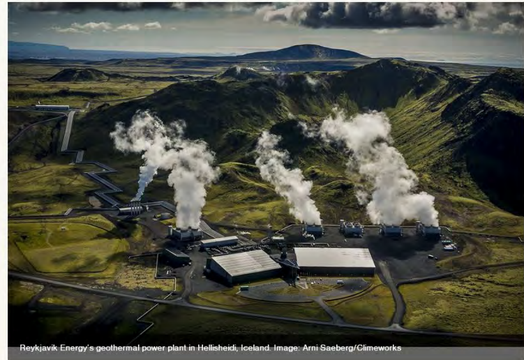
Reykjavik Energy's geothermal power plant in Hellsheiði, Iceland. Image: Arni Saeberg/Climeworks
